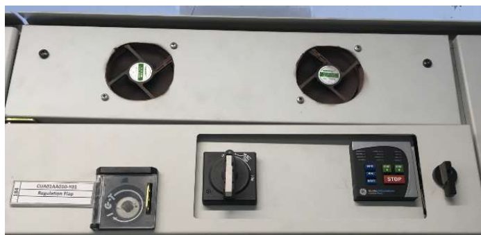
Fig. 19 Best practice fans in each panel (10 drawers/panel).
