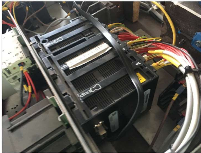
Fig. 14 Do not install self-adhesive tape covering case slots.
