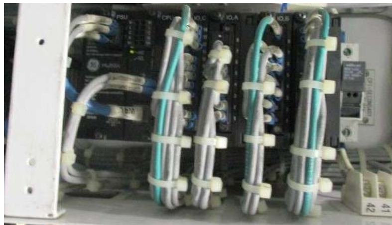
Fig. 4 Example of a proper wiring.
