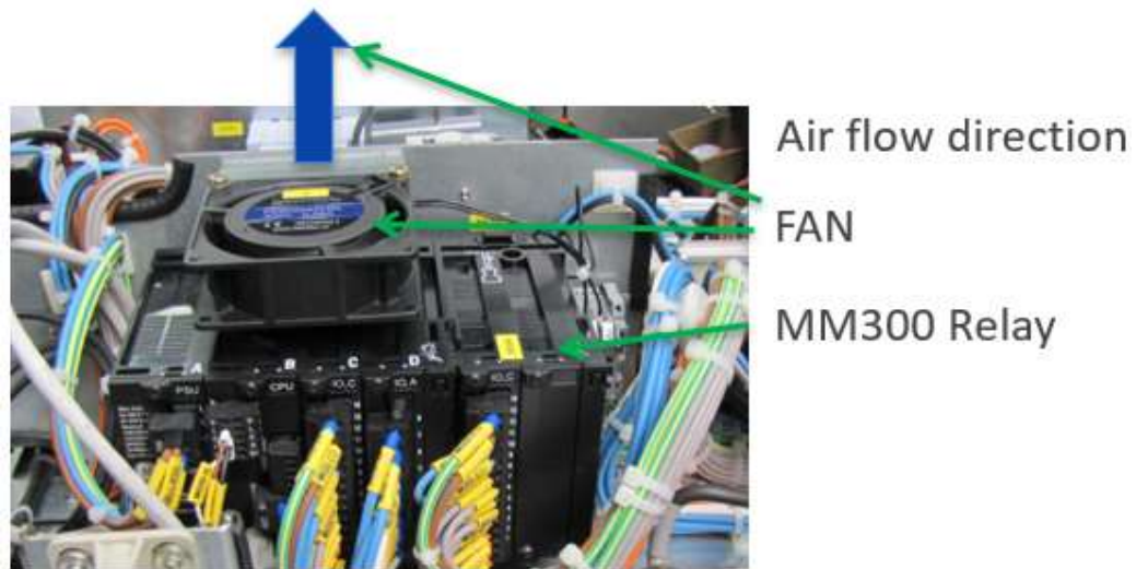
Fig. 18 Example of forced ventilation inside the drawer.
