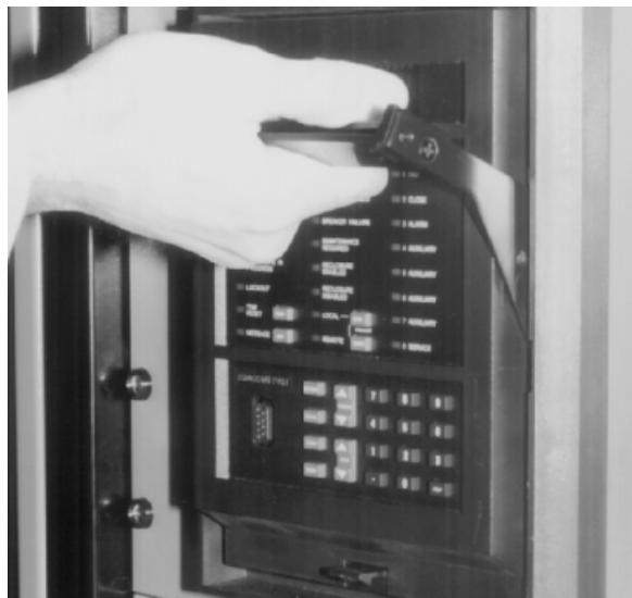
Figure 3-6: ROTATING HANDLE TO STOP POSITION
