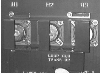
Figure 5. Safety baffle over the fuses.
