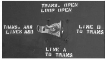
Figure 26. V-blade switch.
