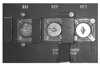
Figure 6. Safety baffle moved from over the fuses.
