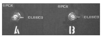
Figure 20. Loop-radial switches.
