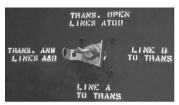
Figure 25. T-blade sectionalizing switch.
