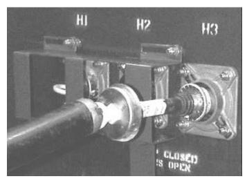
Figure 7. Fuse removal with a hot stick.
