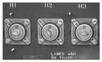
Figure 9. Loadbreak fuses.
