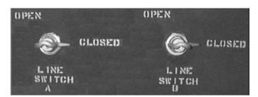
Figure 18. Loop-feed switches.
