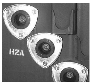
Figure 13. Separable insulated connectors (typical arrangement)..
