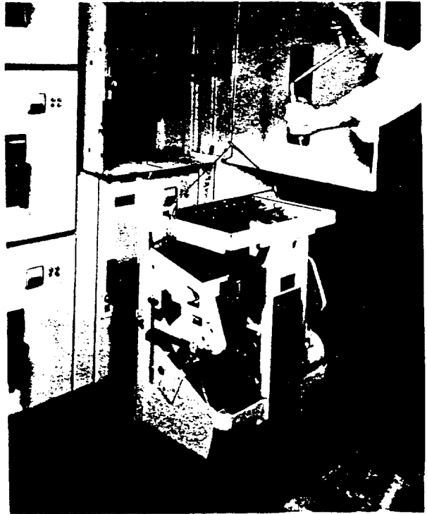
Fig. 17D (8035639) Adjust Cable To Balance Breaker. Proper Ball Must Be Under Cable Eye.
