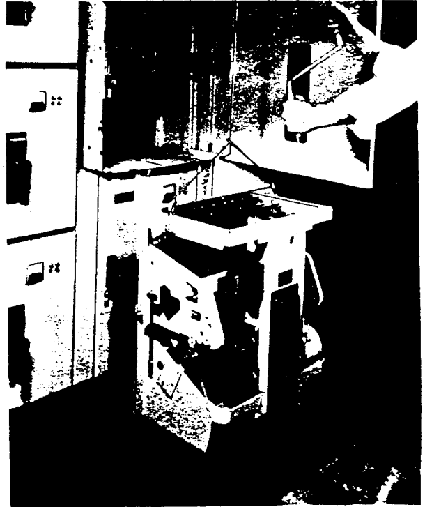
Fig. 17D (8035639) Adjust Cable To Balance Breaker. Proper Ball Must Be Under Cable Eye.
