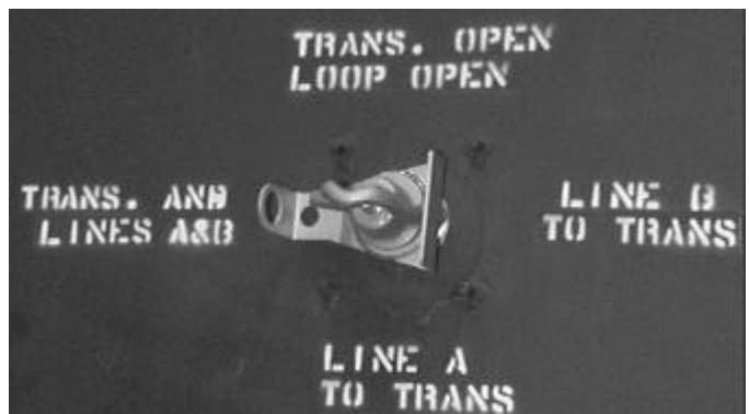
Figure 26. V-blade switch.
