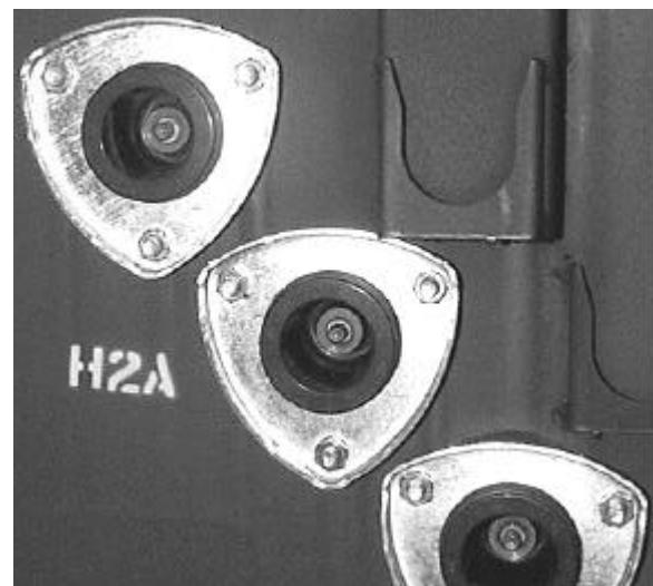
Figure 13. Separable insulated connectors (typical arrangement).
