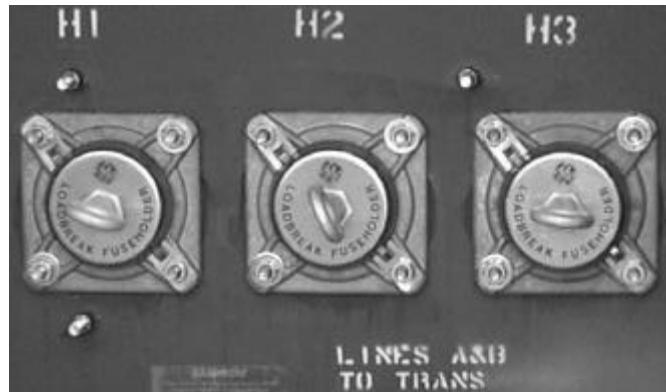
Figure 9. Loadbreak fuses.
