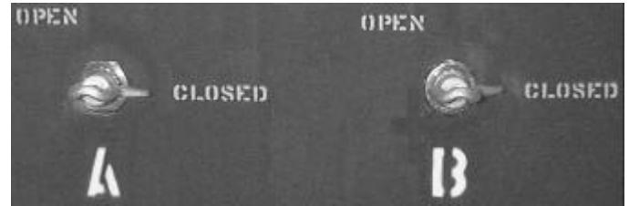
Figure 20. Loop-radial switches.
