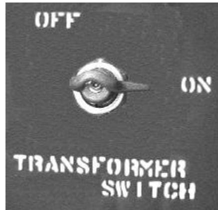
Figure 16. Radial-feed switch.
