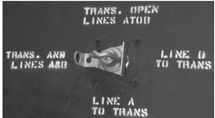
Figure 25. T-blade sectionalizing switch.
