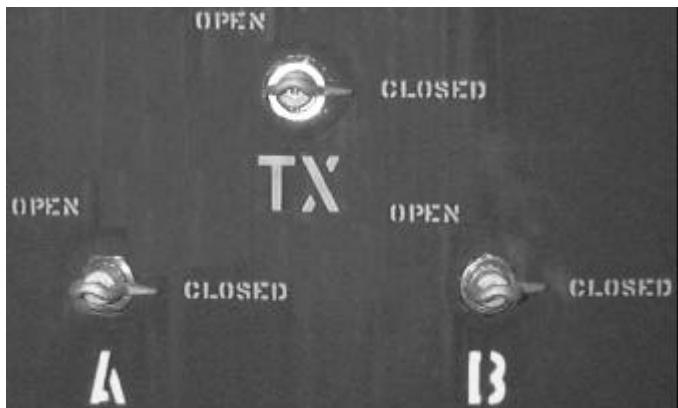
Figure 23. Loop switch with ON-OFF radial switch.
