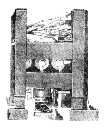
FIG. 7 (8043177) SVC Relay - Side View (Removed from Case)
