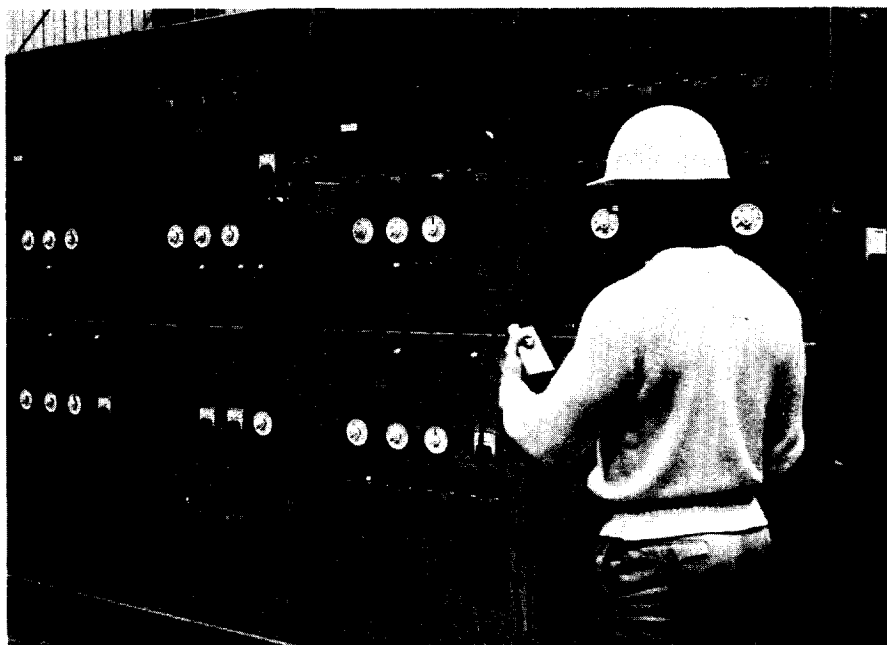
Fig. 11 Remote Racking Operator
