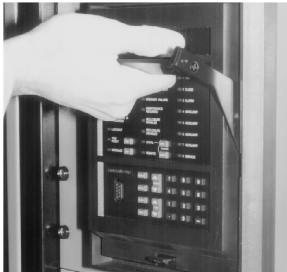
Figure 3-6: ROTATING HANDLE TO STOP POSITION
