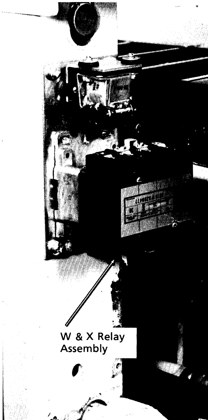
Fig. 14 — W & X relay assembly installed on standard close breaker.
