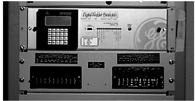
Figure 2-1 DFP200 relay, rack-mounted
